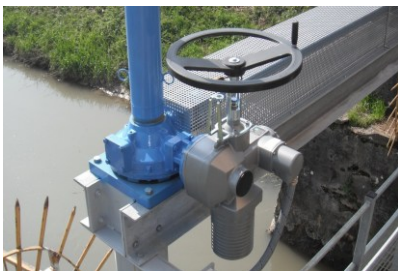
Emergency Kit on AUMA Electric Actuator
