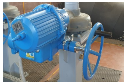
Emergency Kit on DREHMO Electric Actuator
