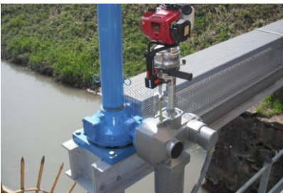
APB/APS tool on AUMA Electric Actuator
