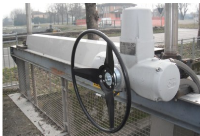
Emergency Kit on BIFFI Electric Actuator
